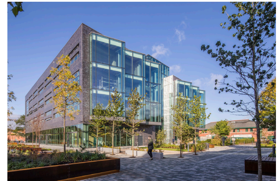
Fig. 29 - Example of potential hard landscaping on plots (Precedent: Bright Building, Manchester Science Park).
