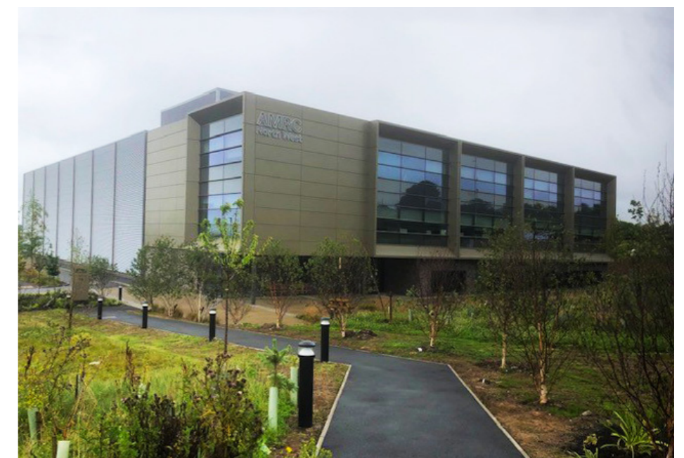
Fig. 30 - Completed landscaping within plots.
